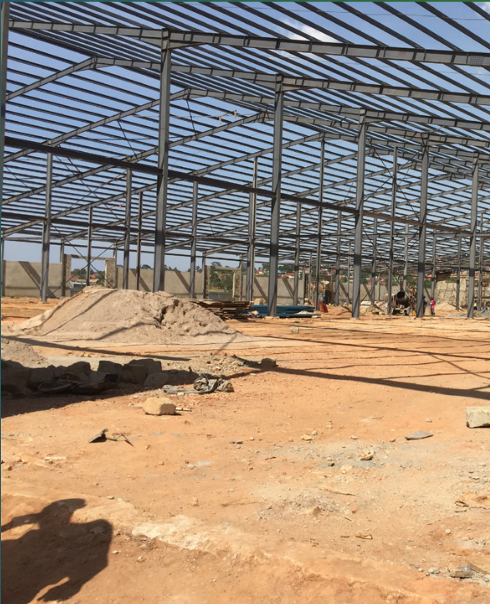
An Inland Container Depo (ICD) with a 1.1 Km railway siding sponsored by Liberty Group to service the Namanve Industrial Park with financing from UDB. Upon completion the project will help decongest Kampala City.
